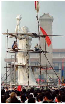
Assemblage of the statue almost finished 29 May 1989
